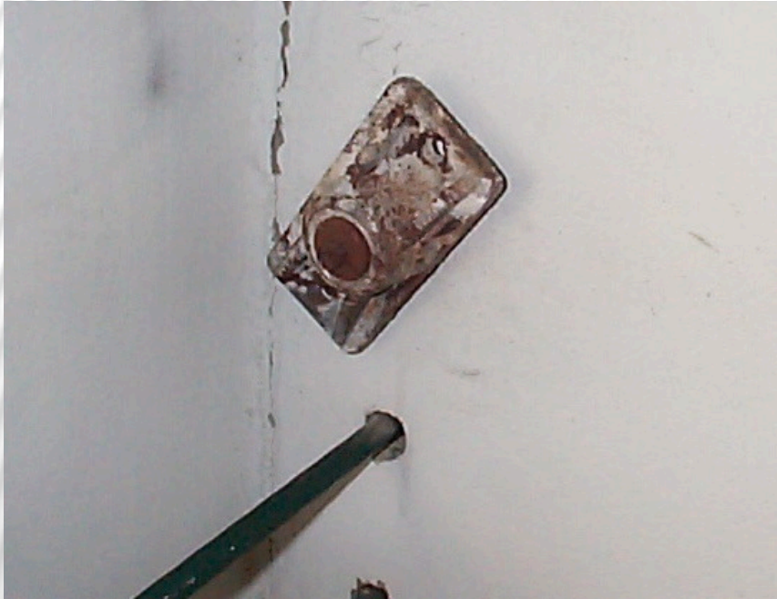
Examples of corroded structural cable anchor and splice.
