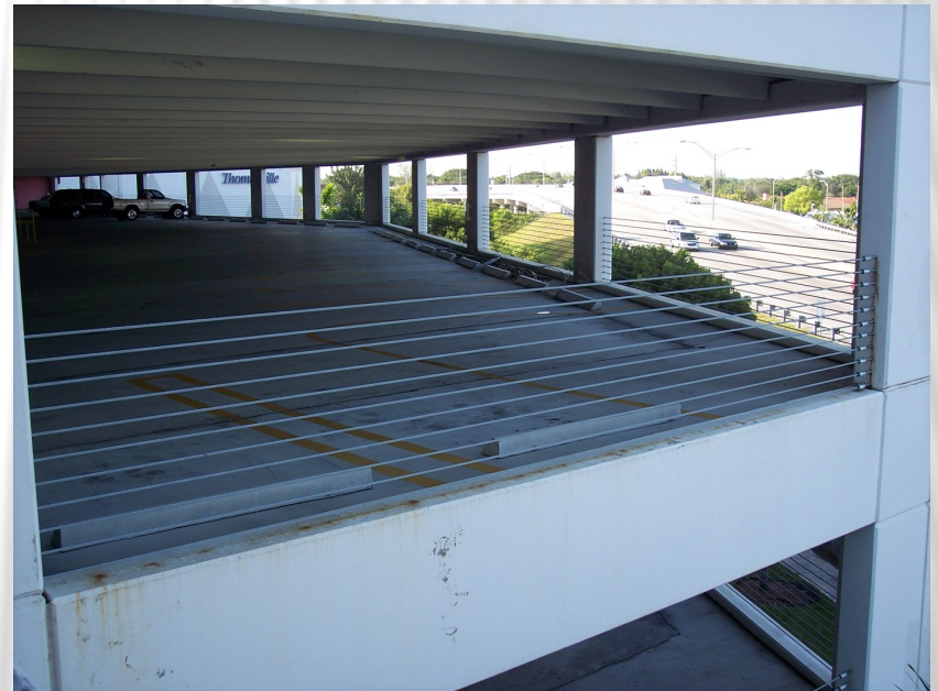
AFTER: New anchors installed and cables replaced.
