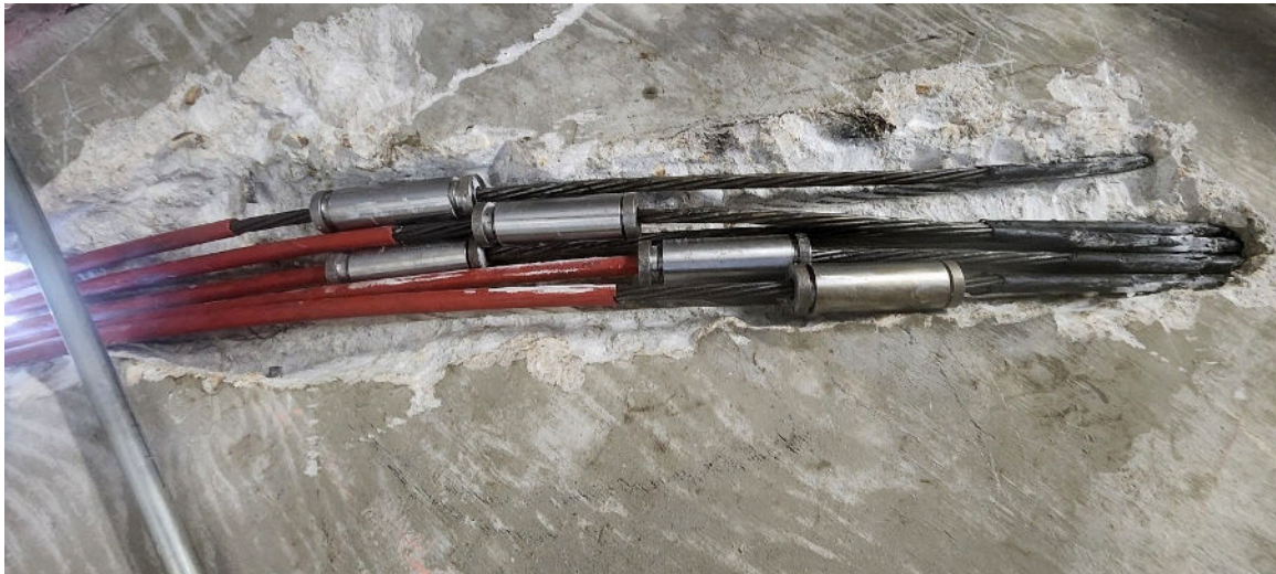
Photo: Installation of these splice couplers within the tendon sweep places an excentric load on the hardware.
