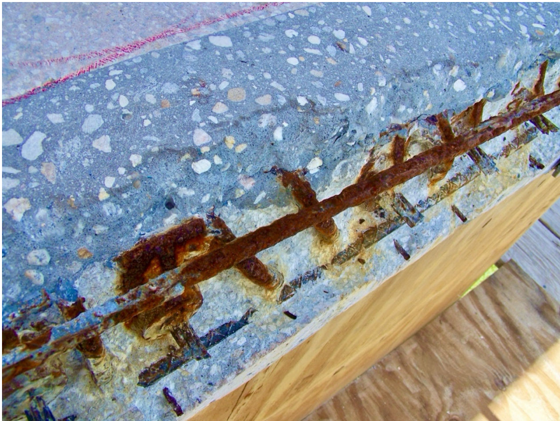
Photo: Old patching material is clearly visible, exposing advanced corrosion of embedded steel.
