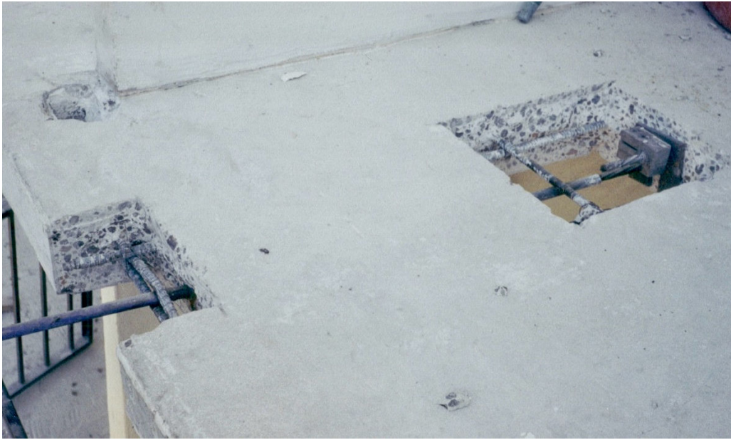
Photo: Shown is a fully excavated slab edge per ICRI requirements with tendon lock-off installed.
