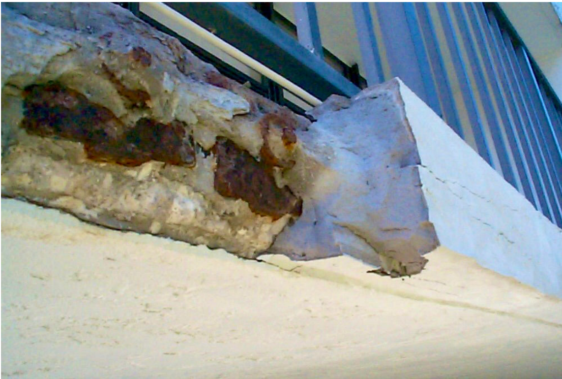
Photo: This failed slab edge patch was applied to the surface of the anchors without fully excavating the damaged area.
