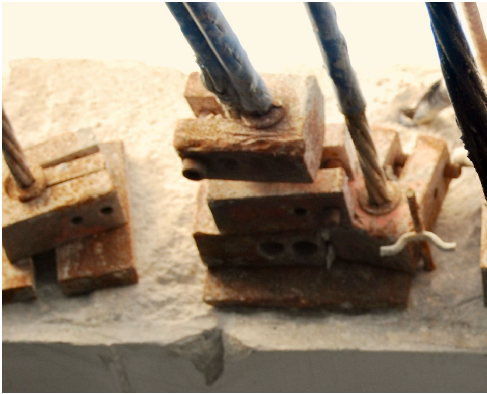
Photo: Bundled cables secured using single cable lock-off anchor that are stacked together.
