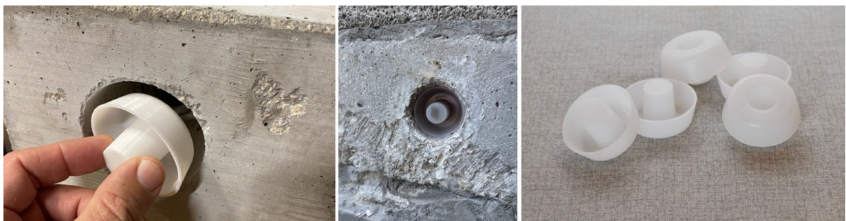
Image 12: The Anchor Pocket Seal before and after installation. ( www.post-tensionproducts.com )
